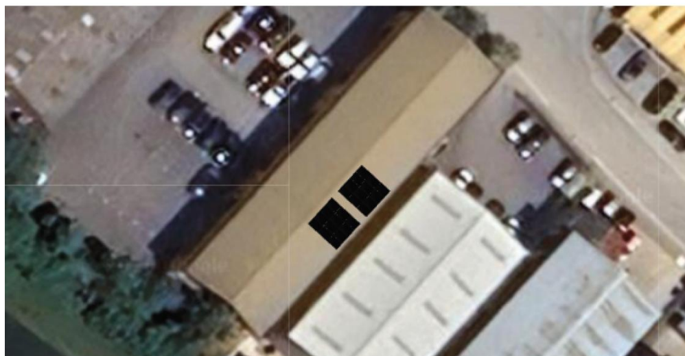
Figure 6: Potential location of rooftop solar PV array
