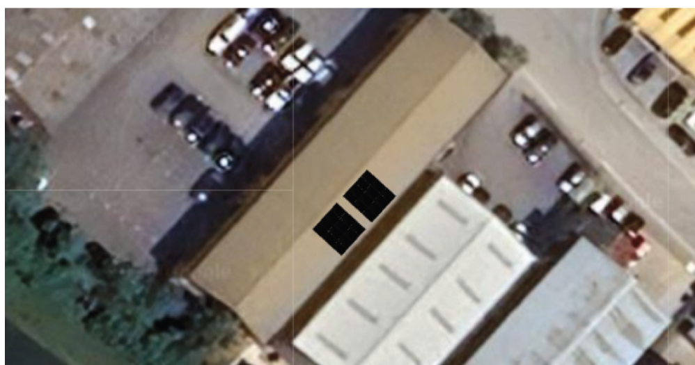
Figure 7: Potential location of rooftop solar PV array
